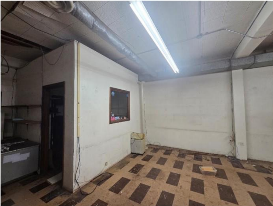
Photo 10: inside demo-ed area, furred out beam colum.
